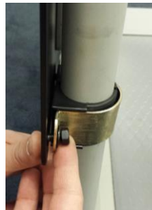
Mounting Plate Bolt Locations
